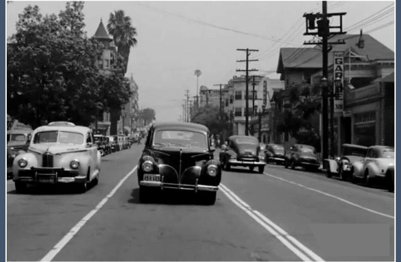
Bunker Hill & Los Angeles Drive (1940)
